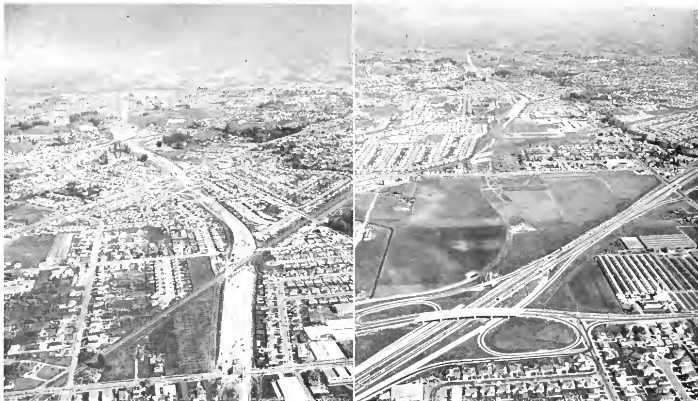
LEFT—Construction operations on Route 228 connection between the Eastshore Freeway at San Lorenzo and Castro Valley. RIGHT—Looking east along location of Route 228 connection from Washington Avenue interchange on Eastshore Freeway to the recently completed Castro Valley Bypass which appears in the distance.
